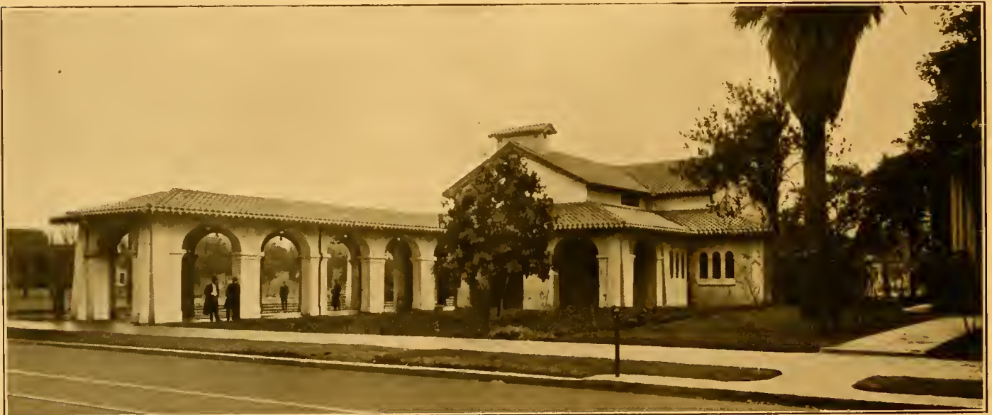
DEPOT OF THE WESTERN PACIFIC RAILROAD, THE NEW TRANSCONTINENTAL LINE
